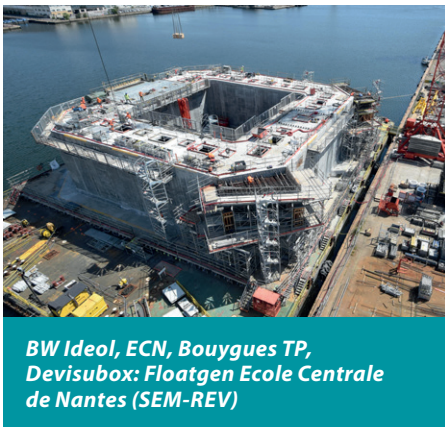
Saitec Offshore Technologies assembly: Port of Bilbao, Spain
